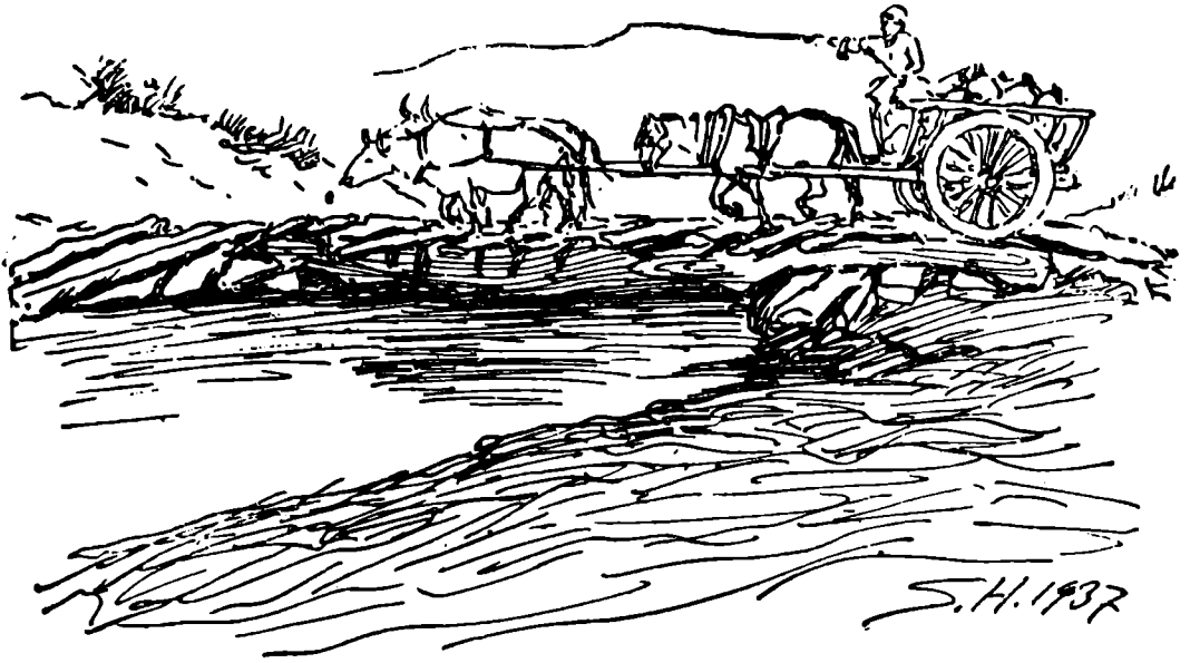
Bridge south of Korla, awkward for motor traffic.
